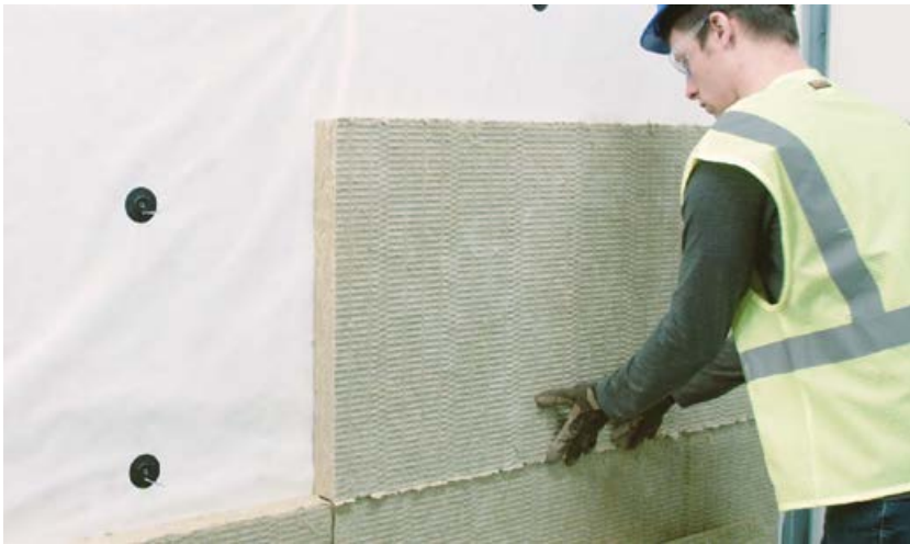
Impaling the insulation over mechanically attached impaling pins.
