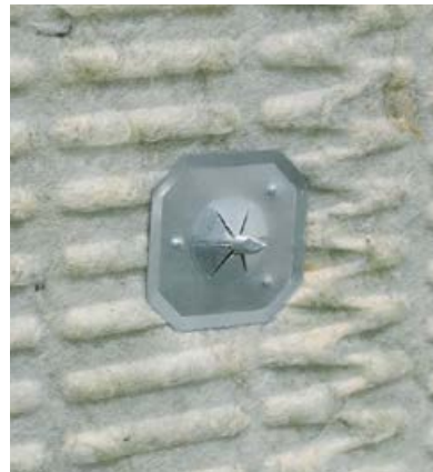
Retaining disc permanently holds mineral wool insulation on a mechanically attached impaling pin.
