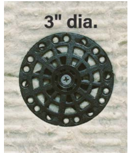
Blind fastening is an option, but be sure to hit the studs and to use a large diameter plastic washer to reduce thermal-bridging and air-barrier penetrations.
